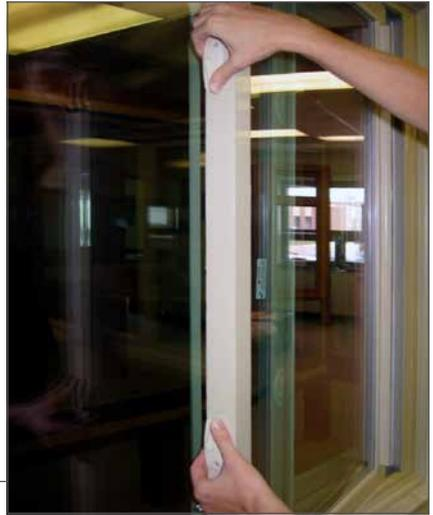
**CAUTION:** Do not attempt to swing in sashes before rotating the cam locks to the “wash” position. Failure to do so will severely damage the windows, creating an issue that is not covered under warranty. Once the sashes are open and have swung inward for cleaning, do not attempt to slide the sashes on the track. This improper operation may cause the sashes to disengage from the window frame causing an issue not covered by the Limited Lifetime Warranty.
