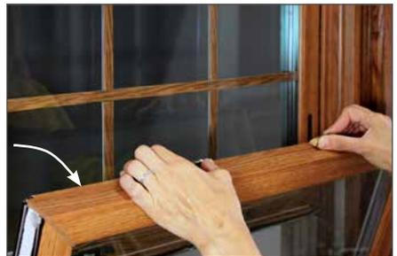
**Push both cam locks to the wash position as you pull the sash toward you to release.**
