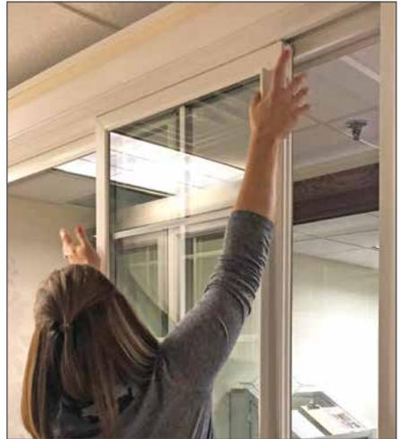
**STEP 5:** Remove the left sash by pulling down on both tilt latches and pulling the top of the sash inward.
