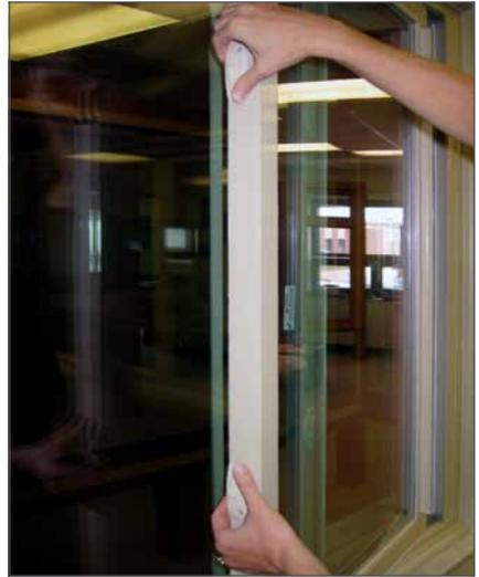
**STEP 2:** Open both sashes so there are equal openings at either end. On right sash, rotate cam locks to wash position and swing in like a door.
