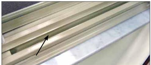
**Water in the track after a rainstorm is normal and will drain out.**
