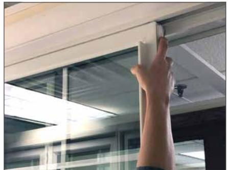
**STEP 3:** Simultaneously rotate the cam lock to the wash position (left) while depressing the tilt latch on the right.
