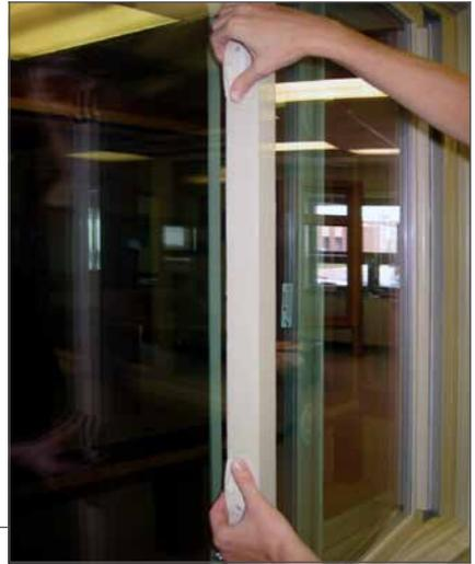
**STEP 2:** Open both sashes so there are equal openings at either end. On right sash, rotate cam locks to wash position and swing in like a door.
