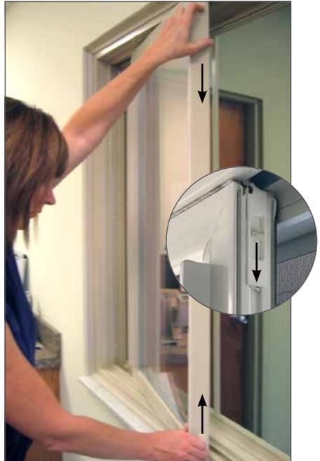
**STEP 3:** Release the left sash by pulling both tilt latches (top and bottom) toward the center of the window and swinging the sash in.
