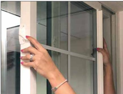
**STEP 3:** Simultaneously rotate the cam lock to the wash position (left) while depressing the tilt latch on the right.
