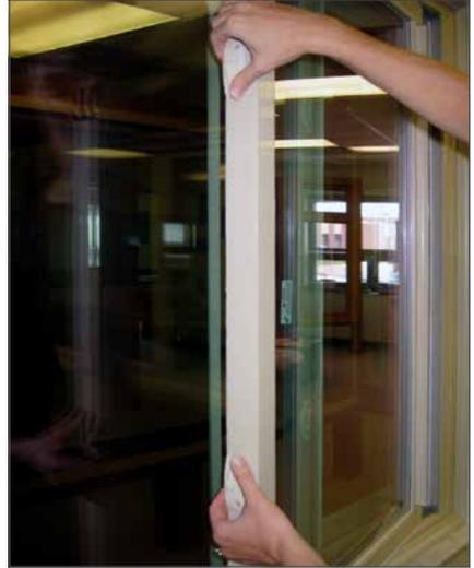
**STEP 3:** The left “keeper” sash has two tilt latches (top and bottom) and no cam lock. To swing in the left keeper sash, make sure it is open several inches. Pull both tilt latches toward the center and hold while pulling the right side of the sash inward with gentle force.
