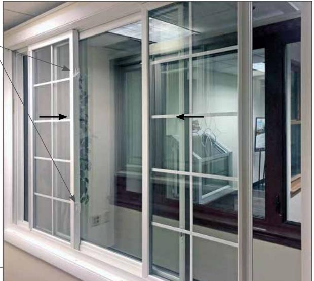
**STEP 1: Unlock and open both sashes so there are equal openings at either end.**
