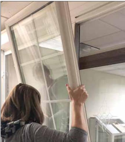
**STEP 4:** While holding the cam lock in the wash position and depressing the tilt latch, pull the top inward.
