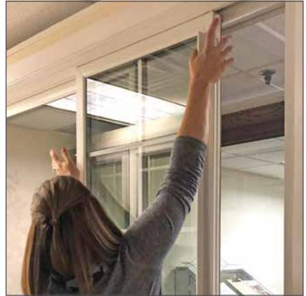
**STEP 5:** Remove the left sash by pulling down on both tilt latches and pulling the top of the sash inward.
