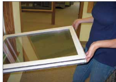
Note: Use care when lowering window sashes, in order to keep balanced and level as you guide to a resting position.
