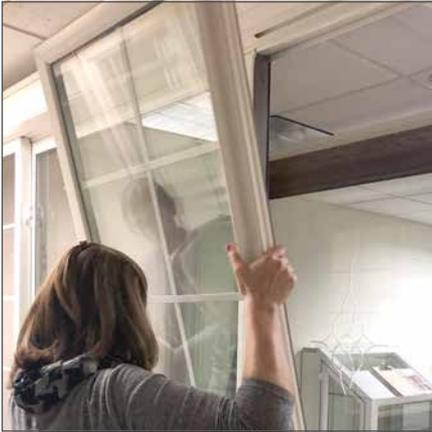
**STEP 4:** While holding the cam lock in the wash position and depressing the tilt latch, pull the top inward.
